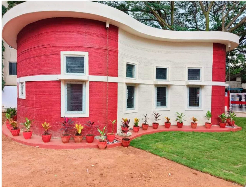
Figure 6 • Printed post office in Bengaluru, India. Reproduced from [38].
