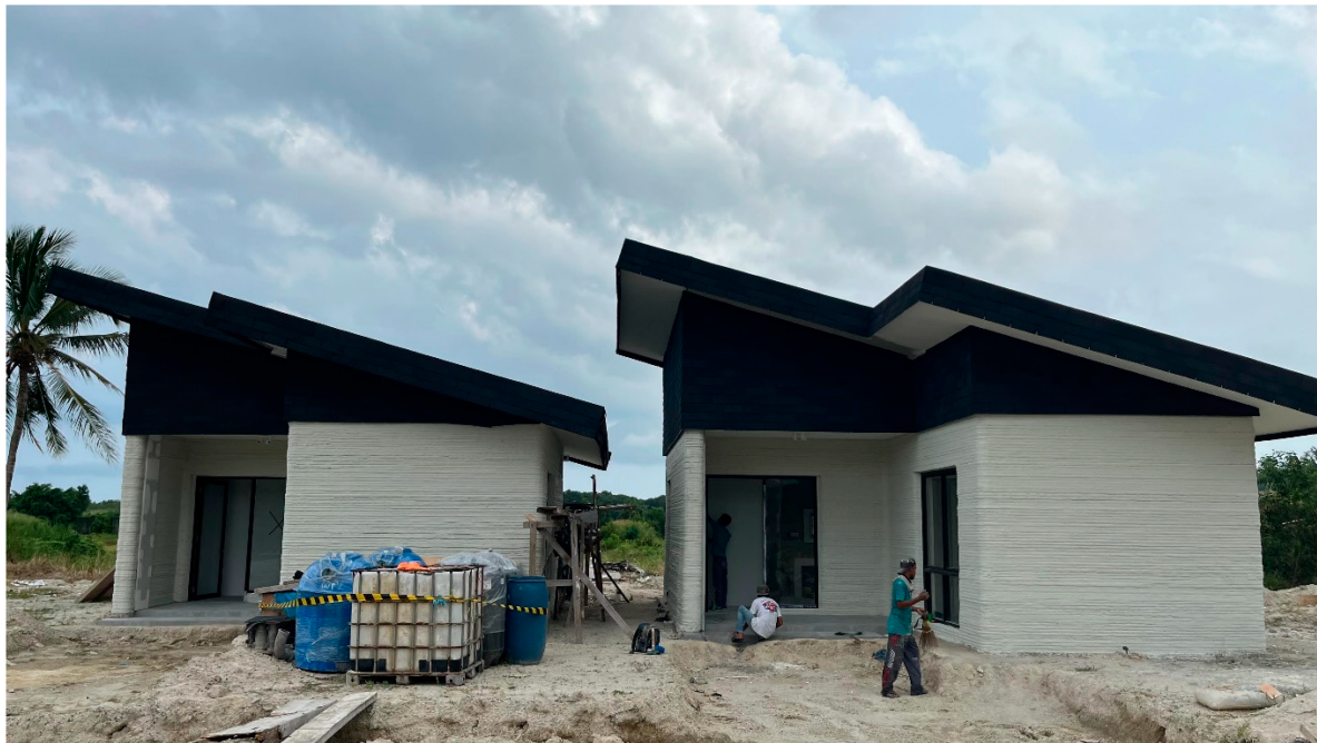
Figure 7 • Three-dimensional-printed house constructed by Modula3D in Bakauheni, Lampung Province, Indonesia (image courtesy of Modula3D, permission granted).
